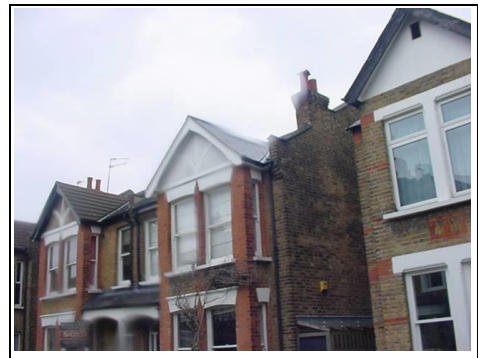
More pointed architecture of a Victorian property
